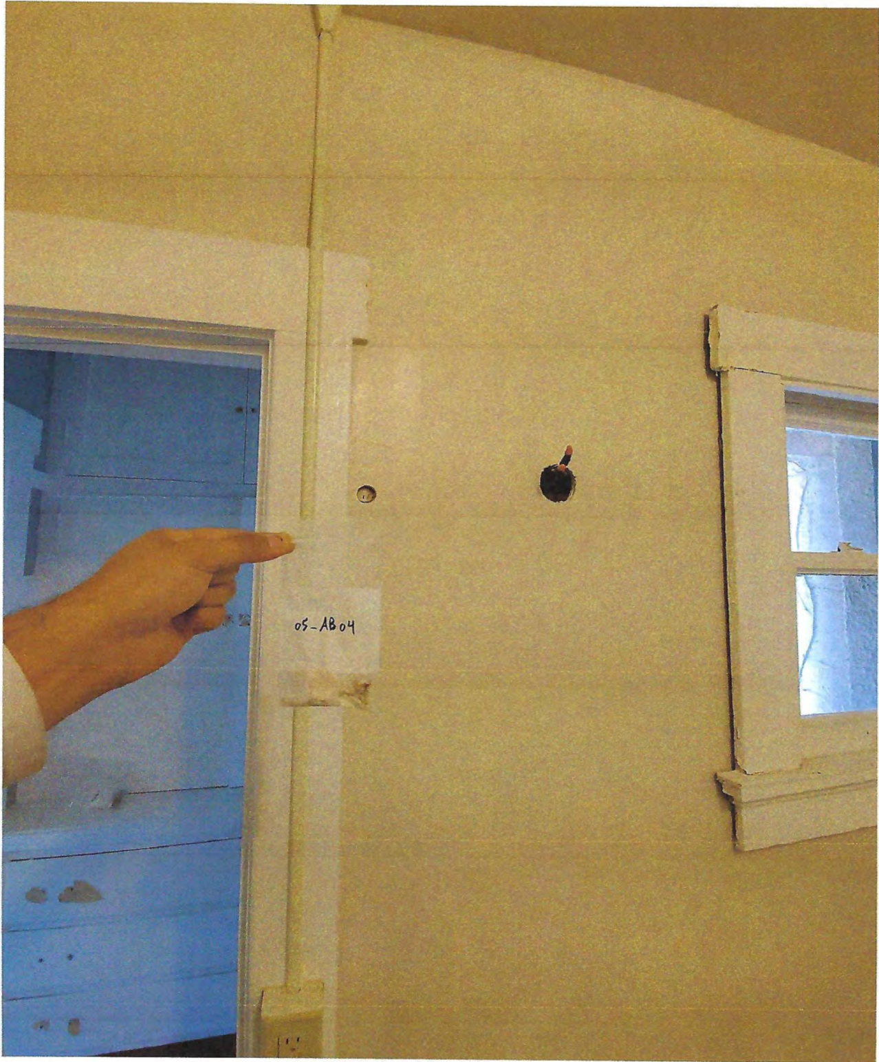
DRYWALL AND JOINT COMPOUND - 2 ND FLOOR
