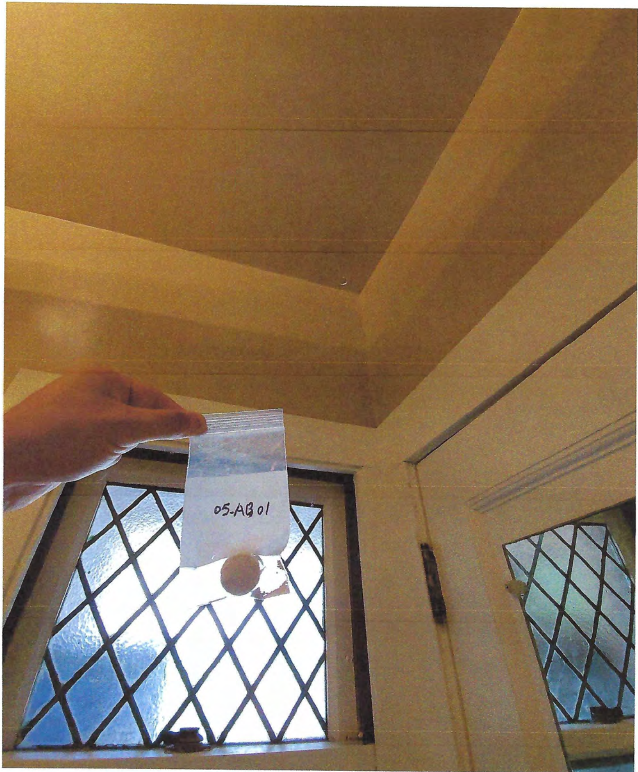
DRYWALL AND JOINT COMPOUND – 1 ST FLOOR
