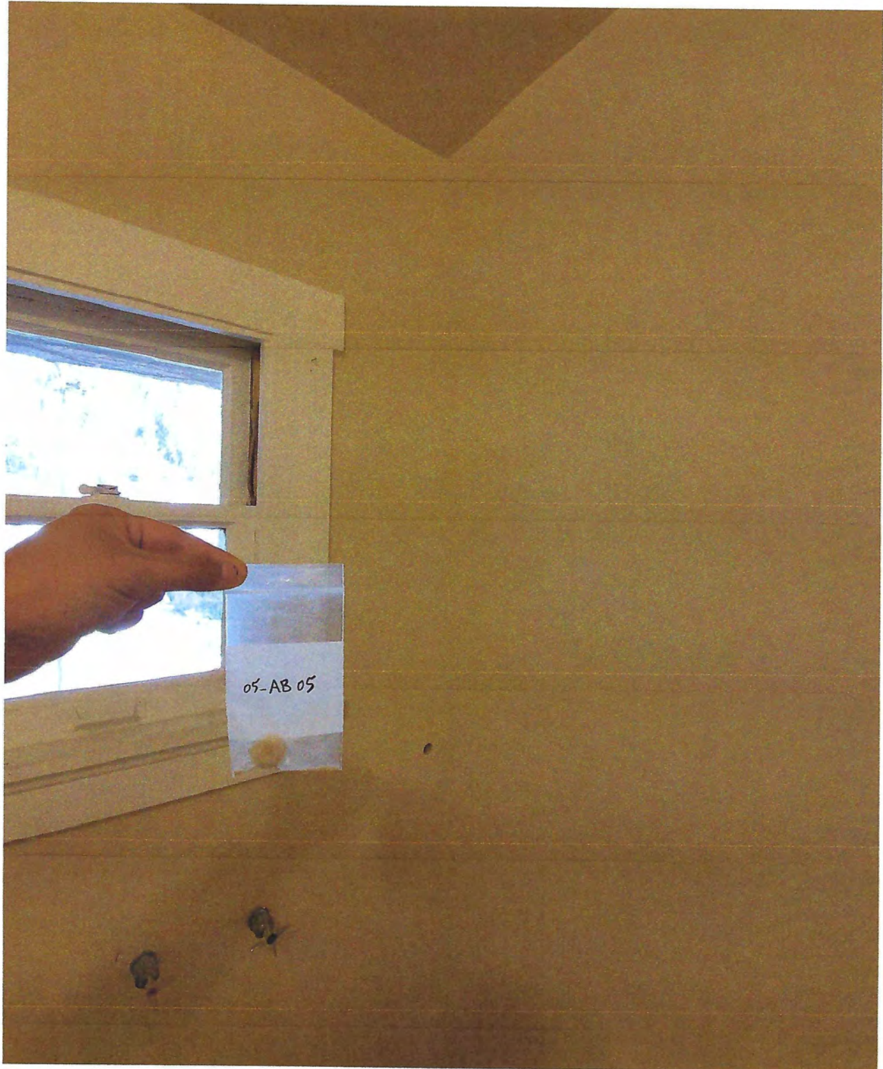
DRYWALL AND JOINT COMPOUND - 2 ND FLOOR
