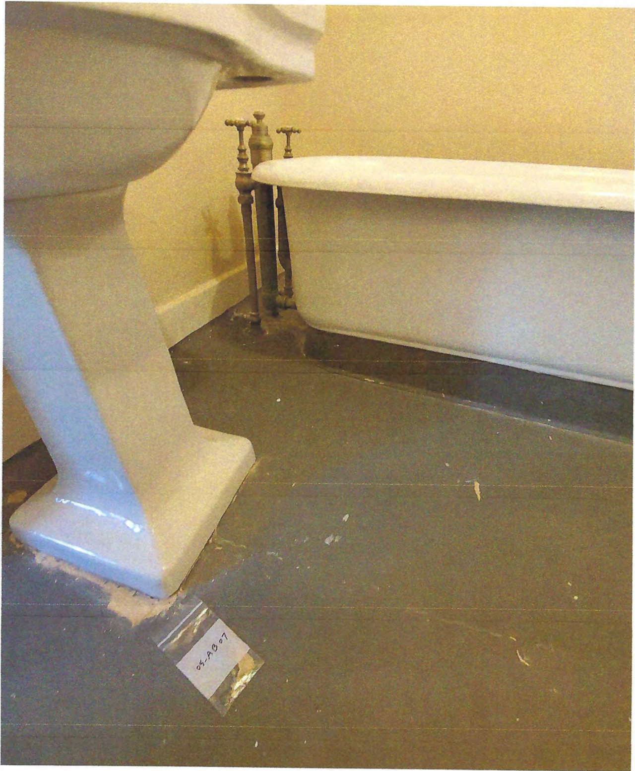
REPAIR SEALANT - 2 ND FLOOR
