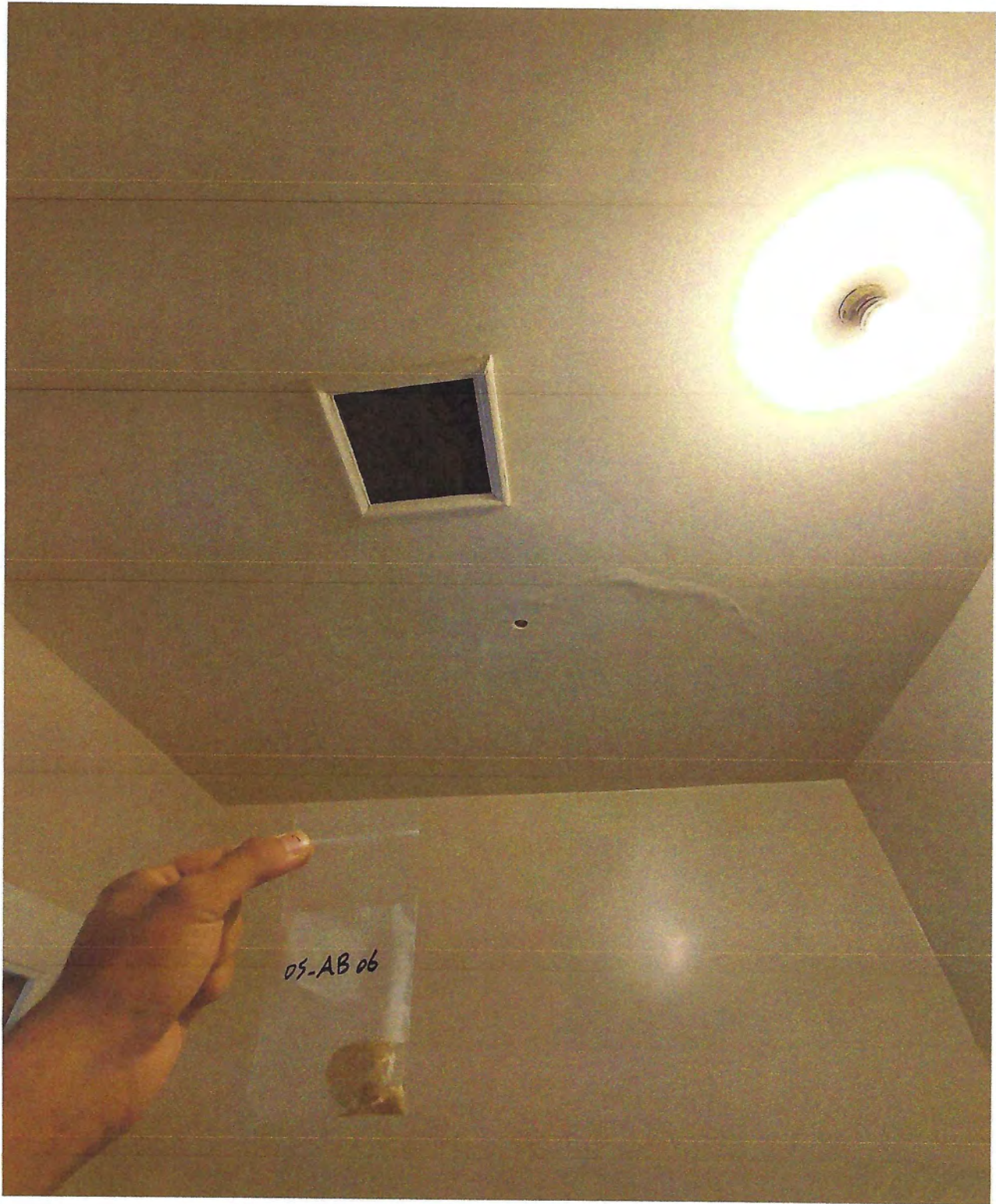
DRYWALL AND JOINT COMPOUND - 2 ND FLOOR
